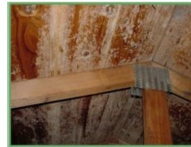
Moldy attic area caused by leaky roof.
